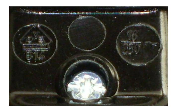
The symbol on the left is the german VDE certification mark (Verband Deutscher Elektrotechniker e. V., Frankfurt am Main/Offenbach) The 614 imprint is of unknown origin, maybe it is the forerunner of the now actual DIN EN 614 (security standards of cables and plugs) or an internal product code of the KOPP company for this specific plug. If you know something about ir, please let us know!
